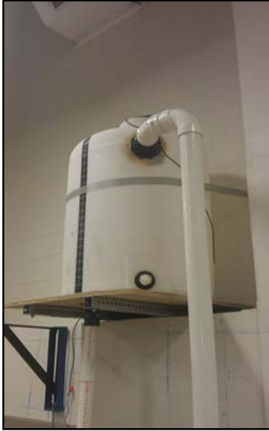
Figure 40: Elevated storage tank
